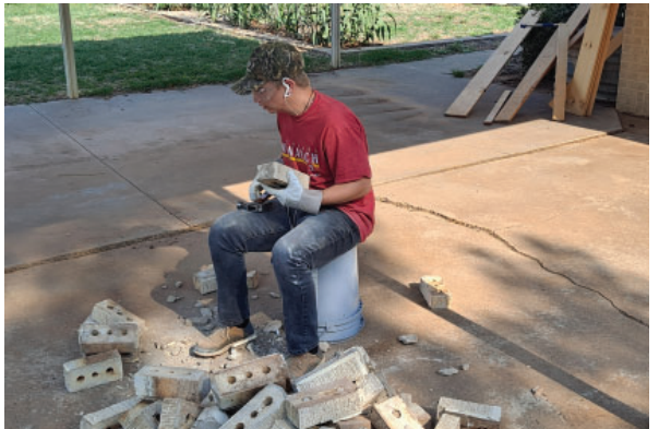
Waste not, want not; cleaning up brick to reuse
